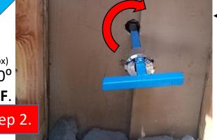
When turning **Water ON** complete steps 1-3 then close all faucets (kitchen sink, bathroom sink and shower) once flow is established.
