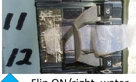
Flip ON/right, water heater breakers handle turning water **ON.**
